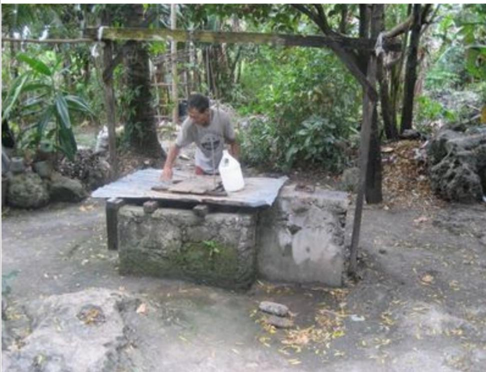
Putting the finishing touches to the new well cap with water pump. A concrete cover will be placed over the well.
